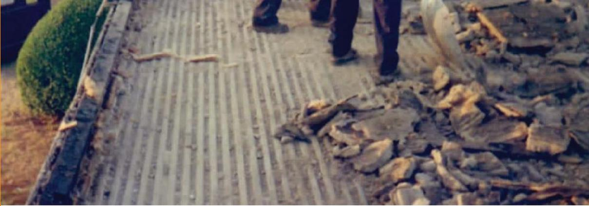
*Failed Lightweight Insulating Concrete*
